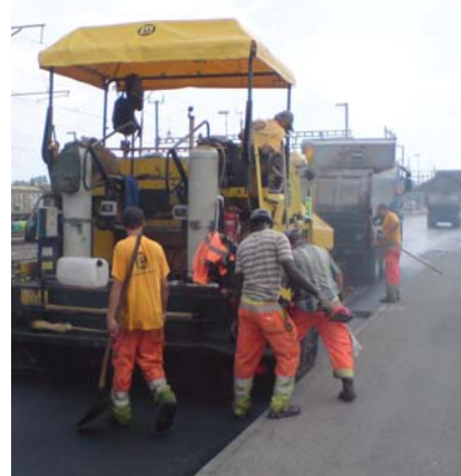
Baustelle in Rothenburg.
