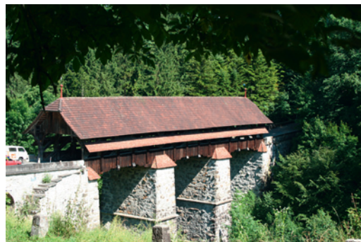
Old bridge across the „Rot“ river
